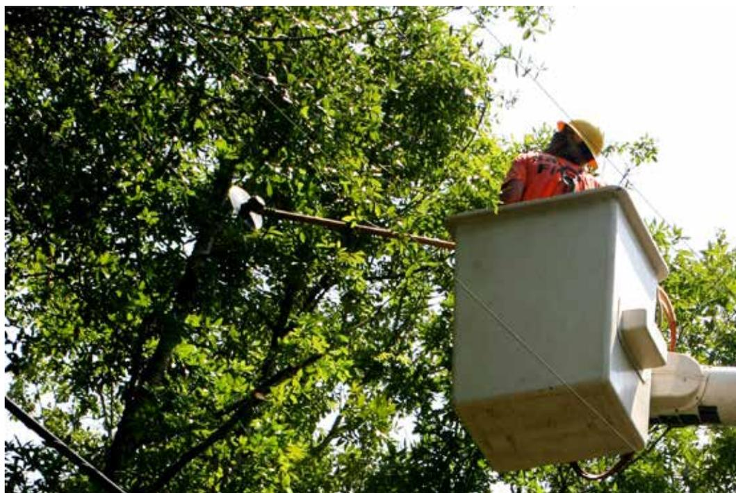
To lessen the threat to lines, CHELCO has increased easements on new overhead lines to 30 feet.
