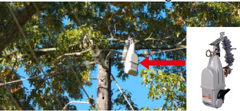
Before the end of 2023, CHELCO began installing automated "TripSaver" reclosing devices along lines in its service area, including Eglin Air Force Base, to help limit the frequency, duration and scope of service interruptions. The programmable devices work like a circuit breaker in a home with the added benefit of automatically re-energizing a power line within seconds to keep power safely flowing to customers.
