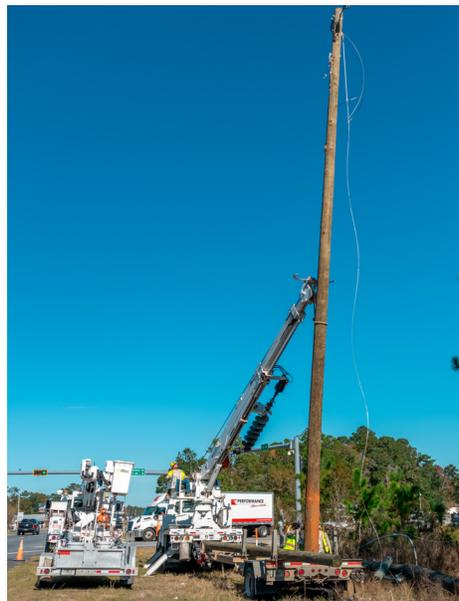
*Today, crews have advanced technology such as the Digger Derrick Truck. Considered a "workhorse," this versatile equipment can dig holes, set utility poles, and lift heavy equipment, such as the nearly 3,000 lb. pole shown here.*
